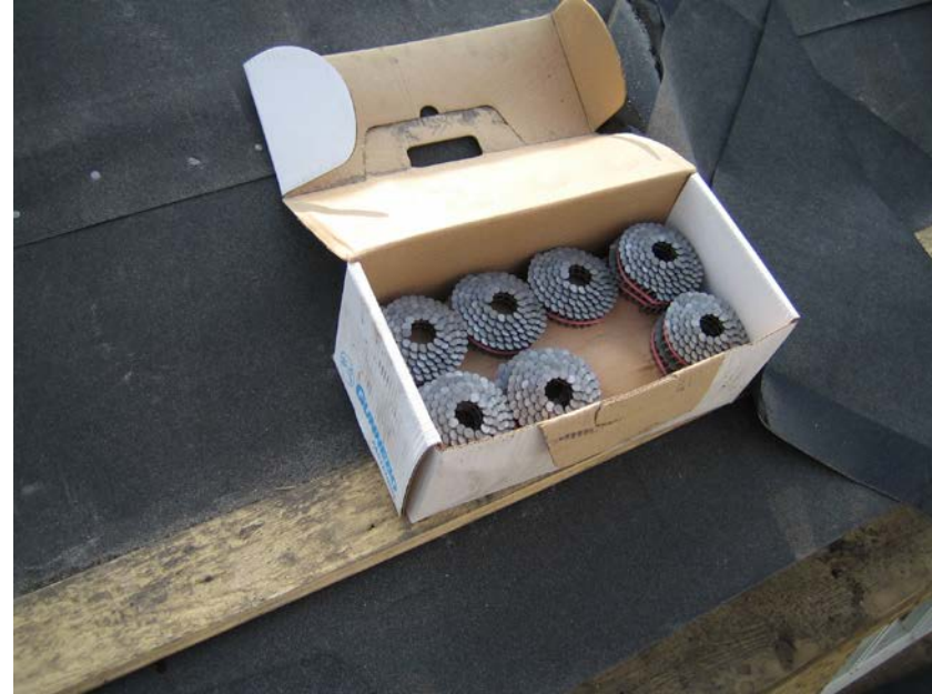
Galvanized roofing paper nails nail in rolls for use in the nail gun.
